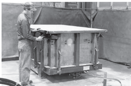
2 Unlatch the corner locking device
