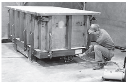
1 Attach the hydraulic pump
